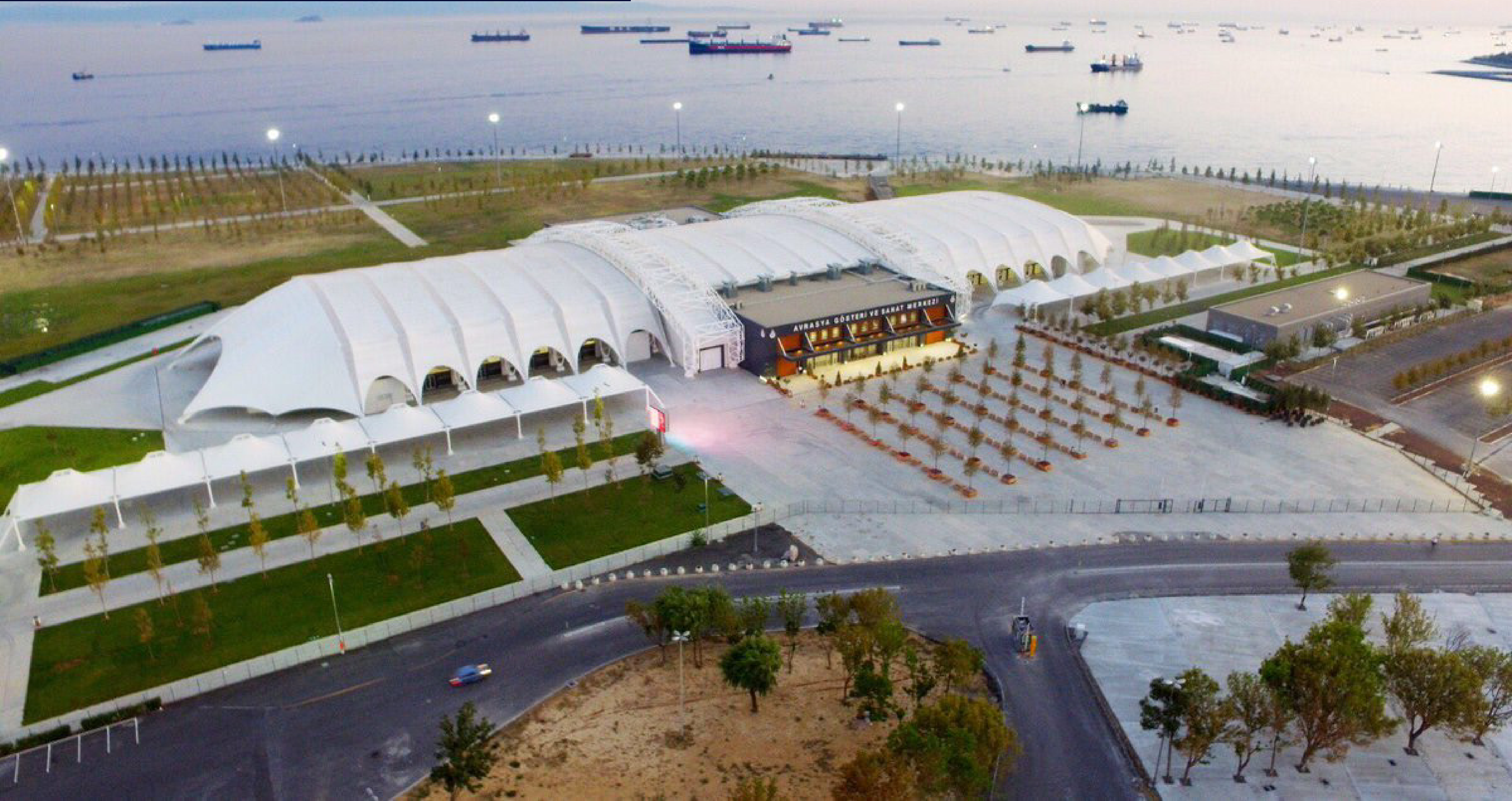
Dr. Architect Kadir Topbaş Performing Arts Center
