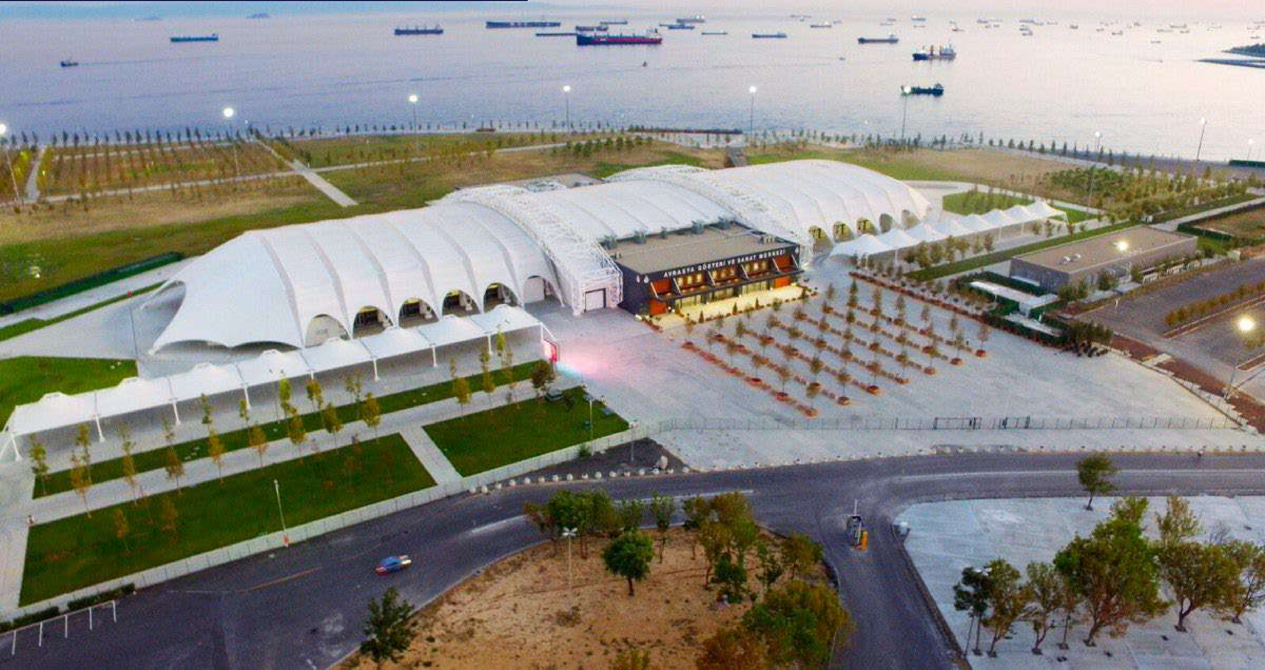
Dr. Architect Kadir Topbaş Performing Arts Center
